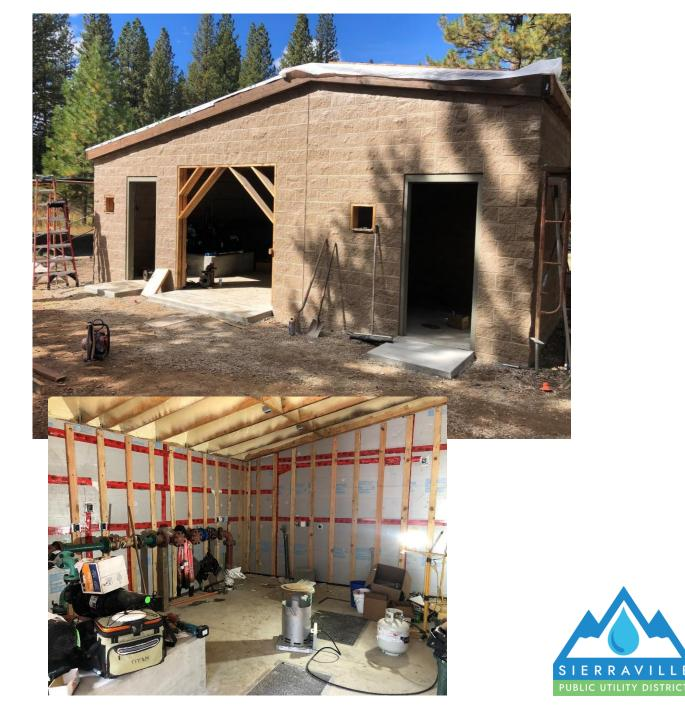
Pump Station equipped with 50KW emergency generator. Fuel source is 1,000 gallon buried propane tank. Funding for generator, automatic transfer switch, fuel tank and related work from Cal OES grant
