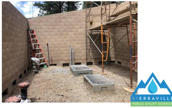
Underslab power conduits, reinforcing and waterproofing before slab pour.
